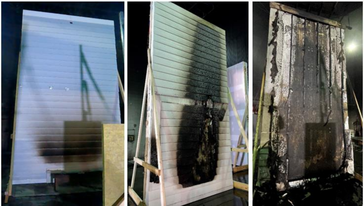
Figure 33 - Side by Side Post-test Photographs from Tests 5-7 of Similar Wall Assemblies with Different Siding - Fiber Cement, Wood Composite, and Vinyl (Left to Right)
